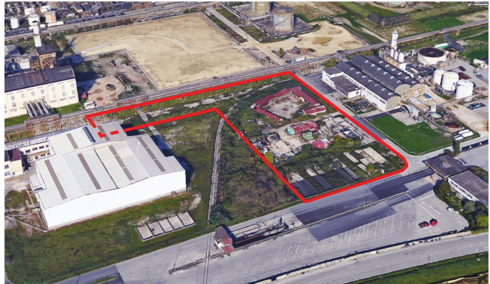
AREA 8.4 - PORTION CTE - DEMI WATER
